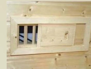
Wooden ventilator sliding grate
